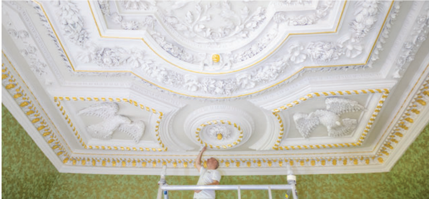
Restoration works on the ceiling at Thirlestane Castle
