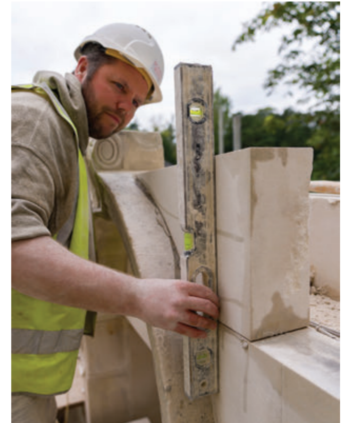
Working on the restoration of screen walls at Woburn Abbey
