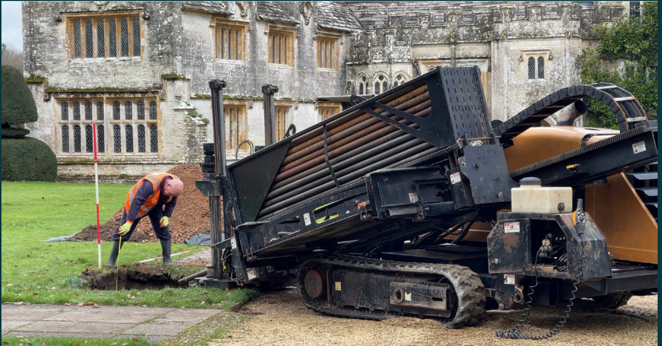
The moling of the underground network of pipes and cables with a directional drill. This method only disturbed a one metre square of historic lawn, which is carefully re-instated by contractors and Athelhampton's gardeners. Photo courtesy of Athelhampton House
