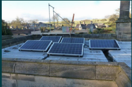
Tissington Hall: 24 Solar Panels on the roof provide electricity for the 400-year-old Hall. This sort of environmentally-friendly and unobtrusive adaptation to a historic building should be encouraged and supported in the planning system.
